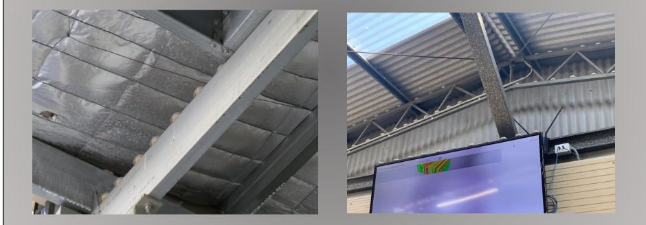
The areas were first cleaned. Dishes of *Bird Fend* were then fitted at 200mm centre to centre, as well as wires utilising the Bird Fend cable tie bases (below left). It is always recommended treating all accessible areas above the targeted area to prevent possible soiling from above.
