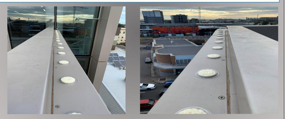
If the ledge is more than 250mm deep, and there is nesting/night roosting in the immediate vicinity of the ledge, two rows of dishes should be applied. Dishes should always be fitted right into the corners of the ledge as birds favour the sheltered corners, then the gels should be installed in a staggered pattern.
